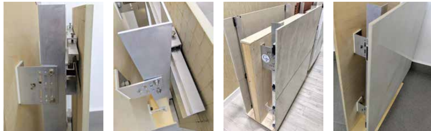
Mockup of Ceramic Panels installed using GIP VECO-A-2000 Substructure System
