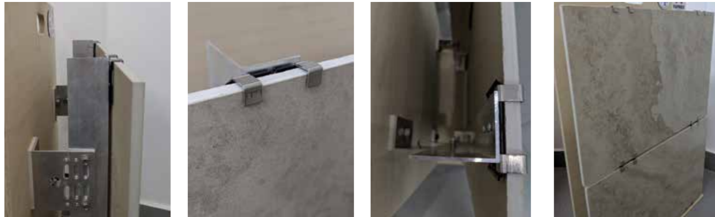
Mockup of Ceramic Panels installed using GIP VECO-A-1020 substructure system
